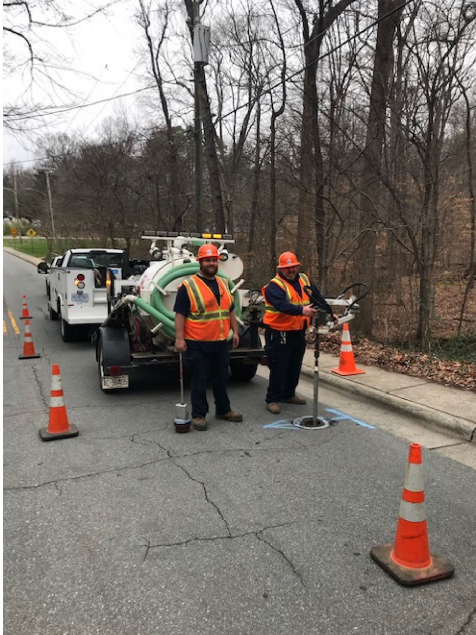
Figure 28: Valve Truck and Valve Crew in Action
